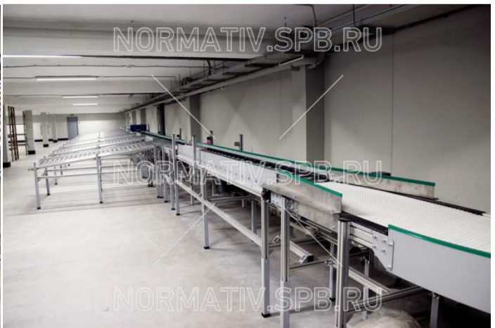
Pic. 3. Ground floor, unloading posts
